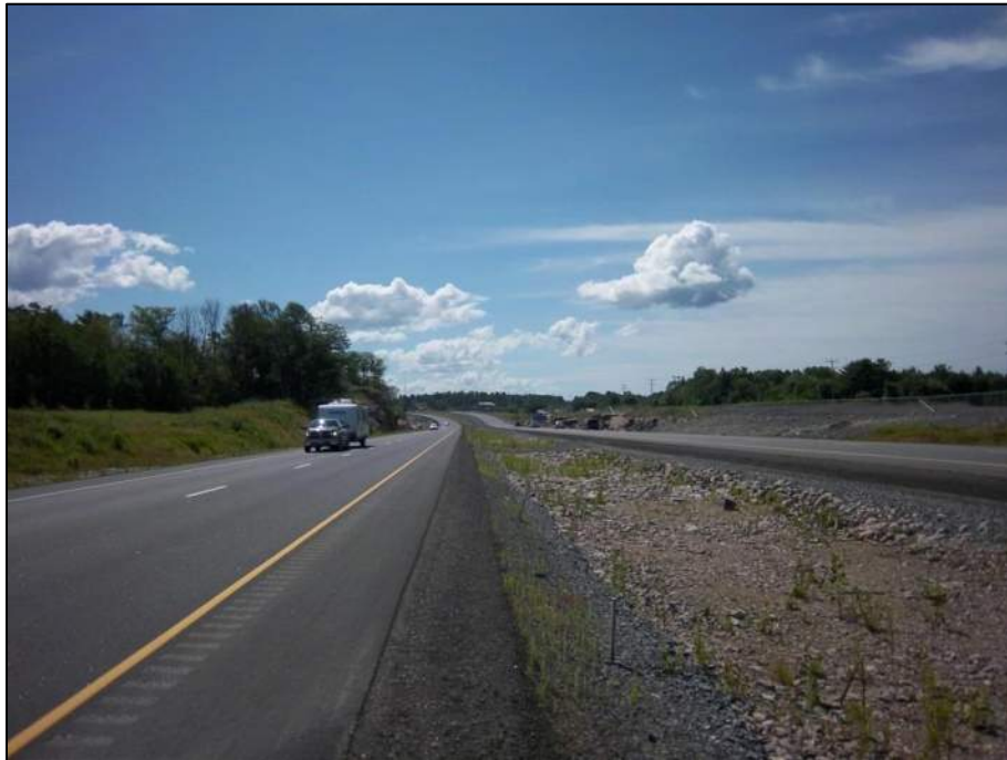
Example of a Four-Laned Section of Highway 11/17
