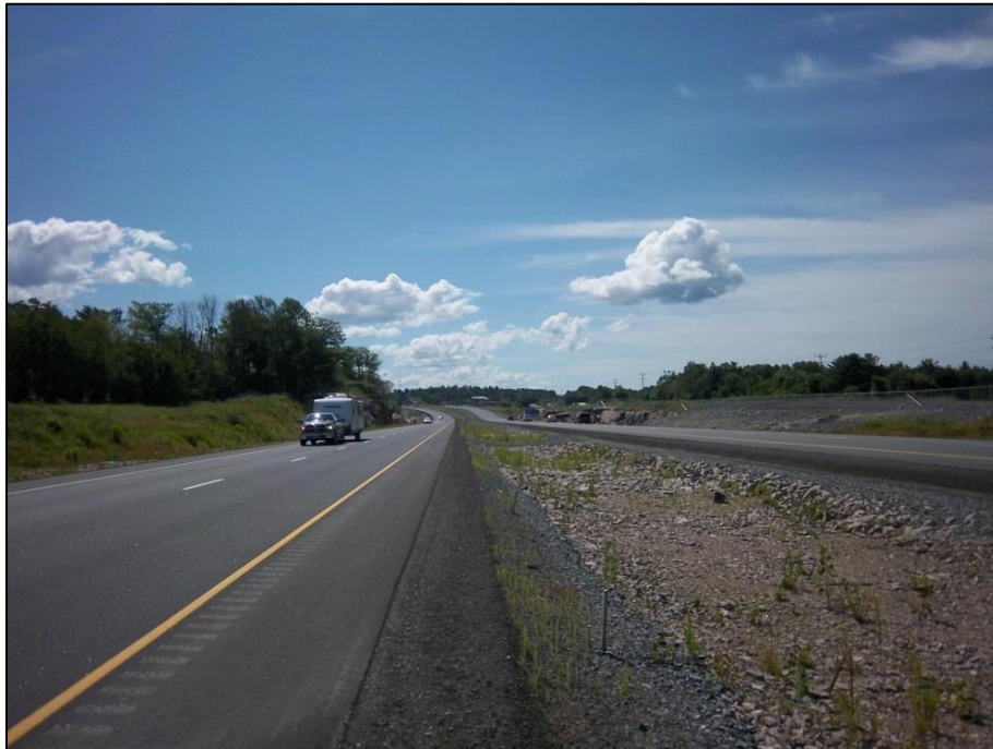
Example of a Four-Laned Section of Highway 11/17
