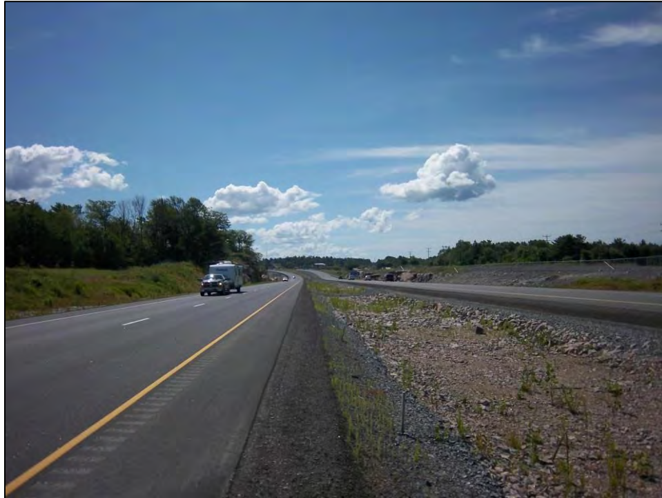
Example of a Four-Laned Section of Highway 11/17
